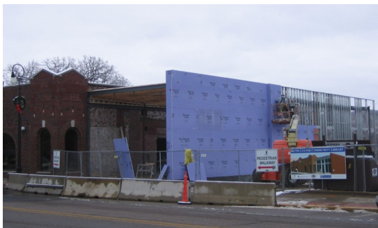
The walls and roof are coming together (December 22, 2011).
